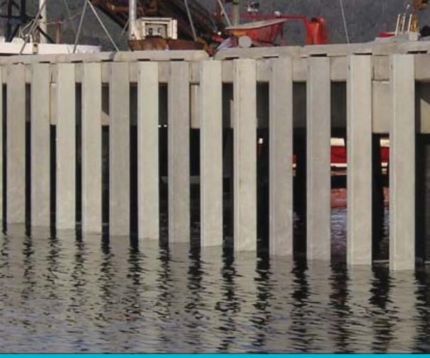
Marine pylons manufactured from recycled plastic (image supplied by Replas)
